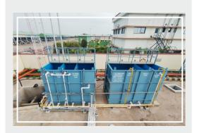
IOCL Jharsugda, Orissa Project - STP Plant Capacity - 40KLD Technology - SBR
