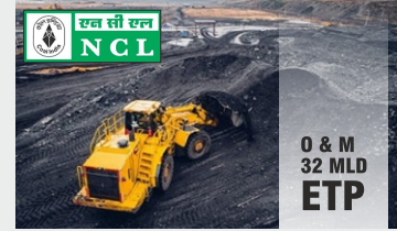
Northern Coal Fields, Bina Project - ETP, Capacity - 32 MLD
