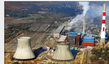
Thermal Power Plant, Sarni Project - STP, Capacity - 2.6MLD
