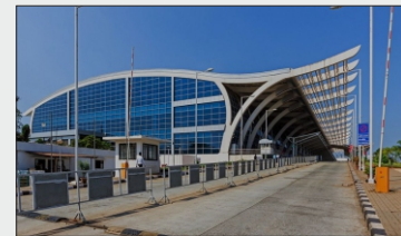
Goa Airport Location, Goa Project - STP, Capacity - 600 KLD
